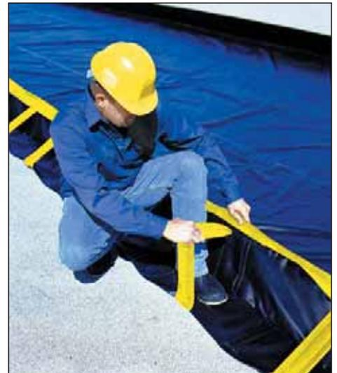
STEP 2: Insert the sidewall struts into their pockets.
