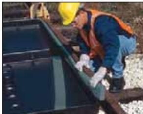
Closed-cell, polyethylene gaskets are then installed to provide a seal between the Pans and rails. (Black gaskets are provided.)
