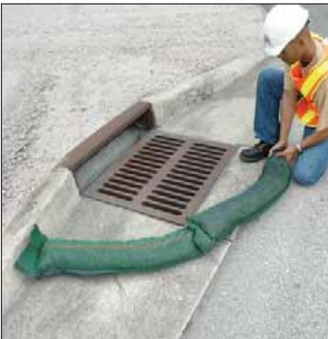
Gravel bags are a basic BMP (Best Management Practice) used to meet regulatory requirements for stormwater and erosion control. The sizes are industry standard and allow the user to fill them up with as much or as little gravel (not included) as the application requires. Different sizes lend themselves to different applications; from drain protection to erosion control at construction sites.
