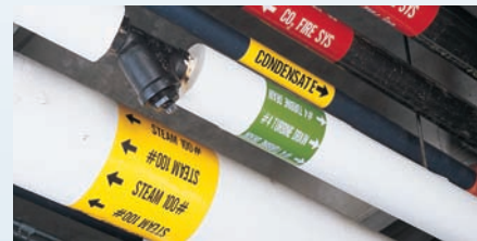
Create roll form pipe markers.
