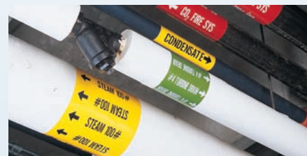
Create roll form pipe markers.
