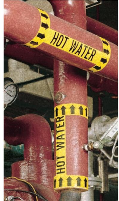
Secure Self-Sticking Vinyl Pipe Markers with Arrow Tape to identify flow direction and reinforce color coding.
