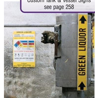
Brady High Performance Pipe Markers are designed for use in harsh environments where there's significant exposure to sunlight, heat and/or chemicals.
