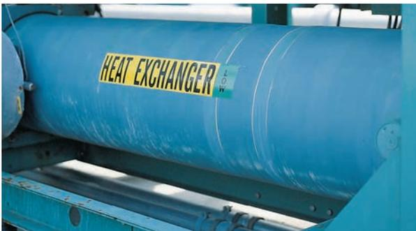
IIAR Component Markers contain the name of the equipment they identify and the designated pressure level.
